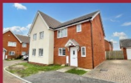
West facing kitchen £349,950 EPC: B
